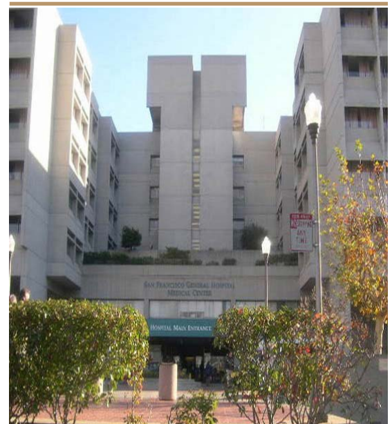
A view of San Francisco General Hospital's main entrance
