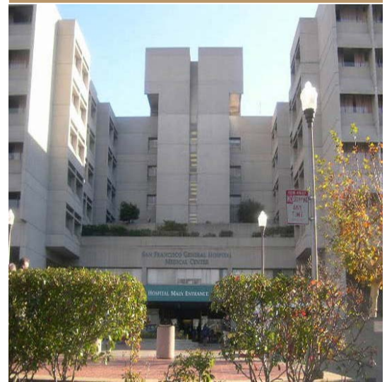
A view of San Francisco General Hospital's main entrance
