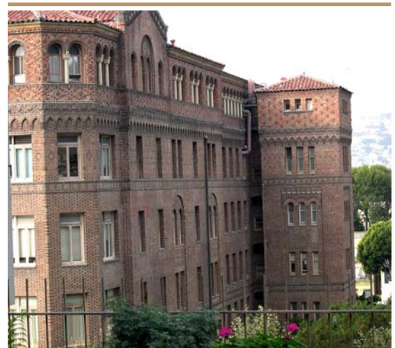
A courtyard view of San Francisco General Hospital's Building 30
